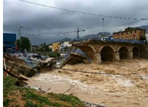
Fig. 2.4.1-7: Images of the bridge affected by the water pressure and the obstruction of its arches. (Source: Citizen platform: Girona River, 2007)
