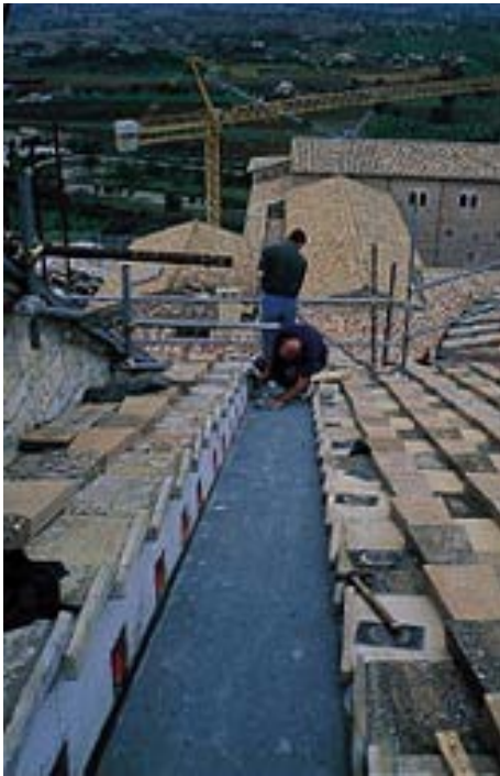
Fig. 1.2.2.-1: Preparing the installation of the SMA devices, (Angeletti P. et al. , 2004)
