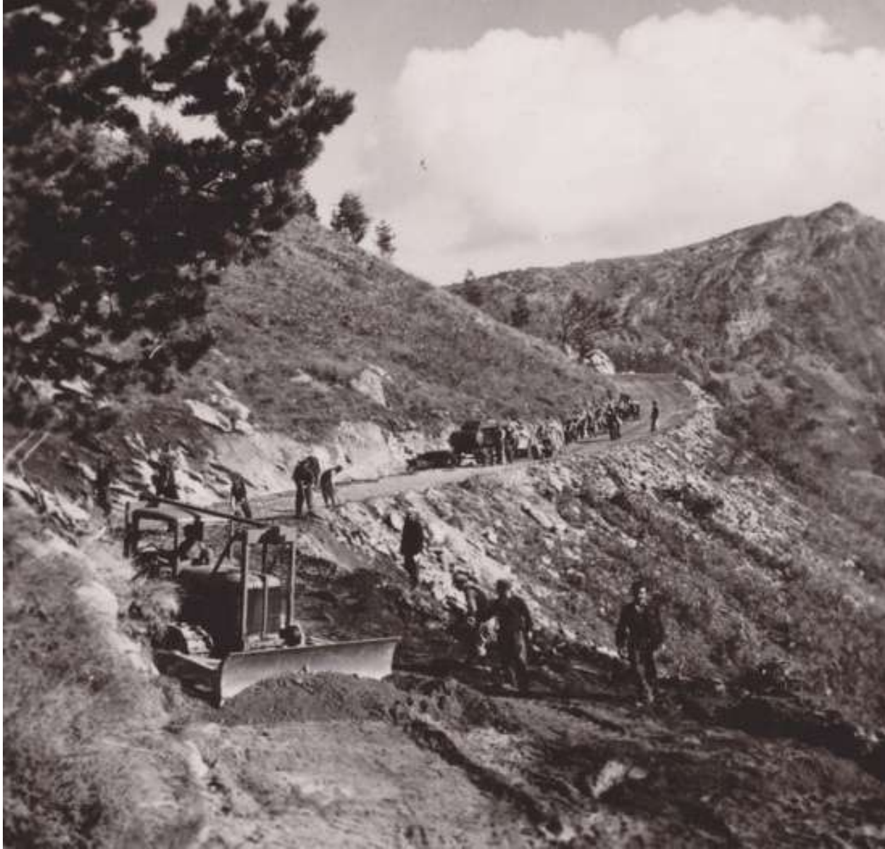
Forest road construction by the GFS in 1950 (Lailias, Serres, N. Greece) Source: Archive of A. Kapetanios
