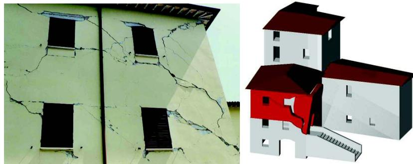
**Figure 7.2.3** This is a masonry building with reinforced concrete ring beams. In this case we can see how important is to achieve the connection between the new reinforced concrete ring beam and the existing masonry.
