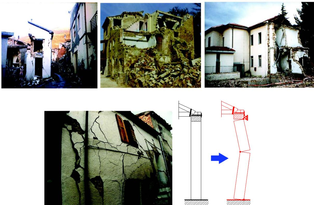
**Figure 7.2.2** In this masonry building it is possible to see a flexural wall failure. There is a good roof-to-wall connection but the middle floor is not connected to the wall.
