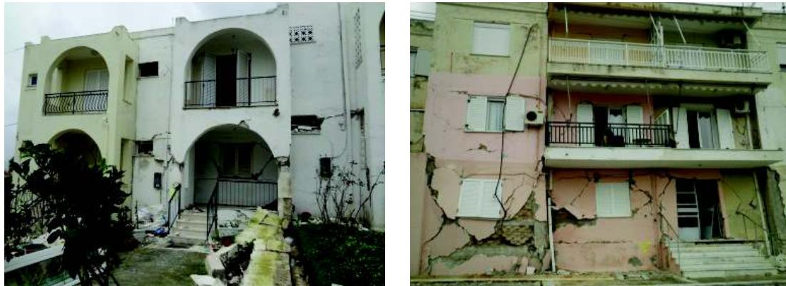
**Figure 7.1.8** Public housing complex heavily damaged buildings in Lixouri (EPPO, 2014)
