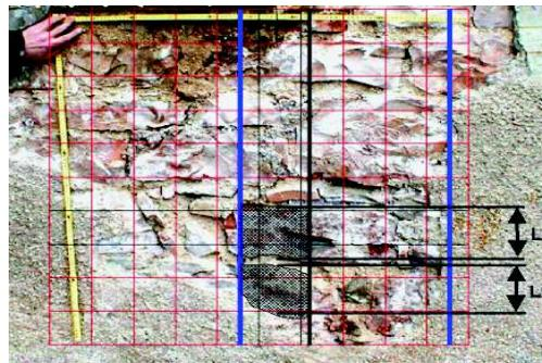
**Figure 7.2.15** Conventional evaluation of the effectiveness of connection between perpendicular walls. The removal of plaster took 20 minutes.
