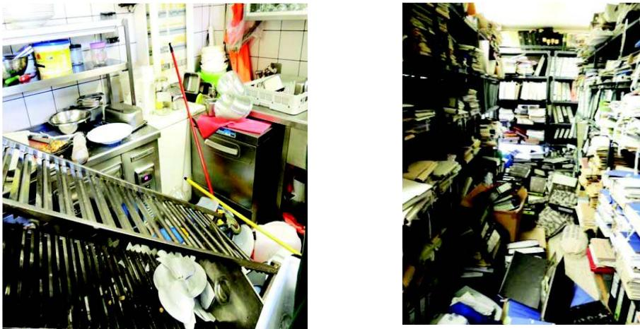
**Figure 7.1.12 Non structural damage: Lack of seismic protection for rolling restaurant shelves, lack of shelving restraints and lack of support for ceiling tiles and light fixtures (GEER/EERI/ATC).**
