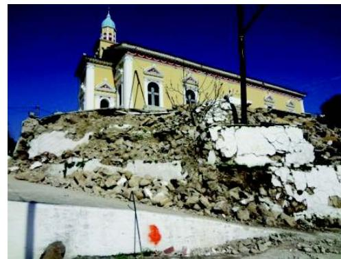
**Figure 7.1.4** Failures at the stone retaining wall in Havriata village (EPPO, 2014)
