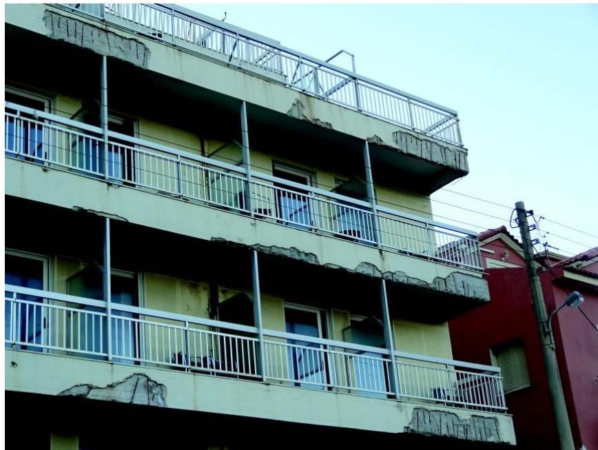
**Figure 5.3** Damaged building at 2014 Cephalonia Earthquake in Greece (EPPO)
