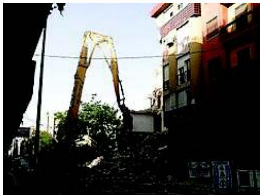
**Figure 7.4.4** Demolition of a building at Santa Fe Jerome, a common scene in the months following the earthquake (<https://commons.wikipedia.org>)
