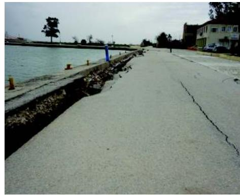
**Figure 7.1.6** Damage at Lixouri port
