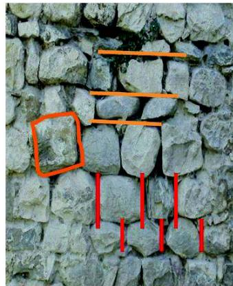
**Figure 7.2.6 Example of the evaluation of the quality masonry in a qualitative way (Source Angeletti, Borri, Longhi, Nasini, Severi (2004) "The law for seismic prevention in Umbria, Italy")**
