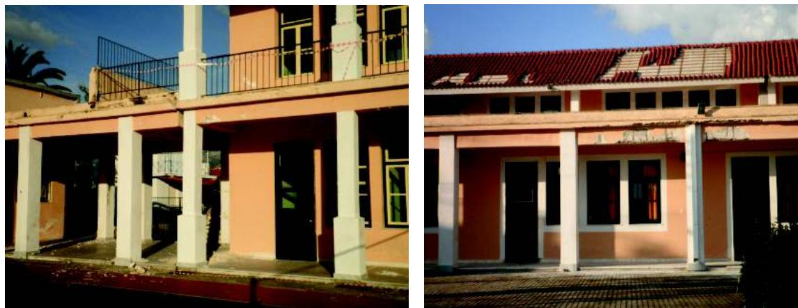
**Figure 7.1.9** "Petritsio" high school, in Lixouri, suffered minor-moderate damage from 2014 earthquakes (EPPO, 2014)
