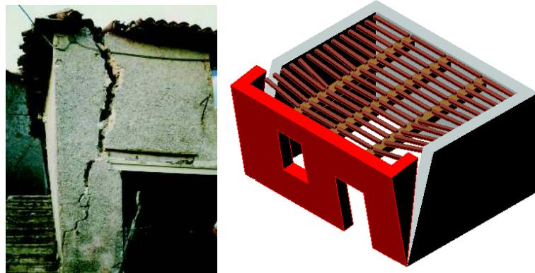
**Figure 7.2.4** In this masonry building it is possible to see the overturning of the wall caused by a poor connection of the roof to the wall.
